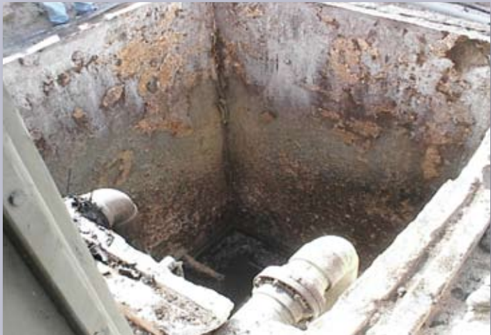
Exhibit 2: Examples of Utility Renewal and Replacement Needs
